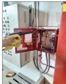
Photo 2.5 Cleaning Control Jockey Pump Cabinet
