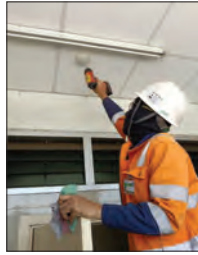
Photo 4.6 Check and Test Heat Detector.
