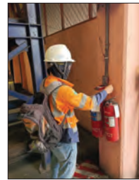
Photo 4.11 Check and Test Manual Pull Station.
