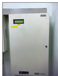
(A). Fire Alarm Control Panel. (FACP)
