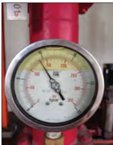
Photo 5.1.23 Pressure (Discharge 132 PSI).
