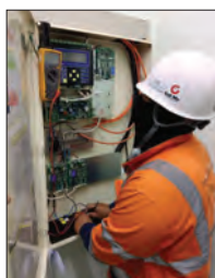
Photo 2.1.2 Check Backup Battery.
