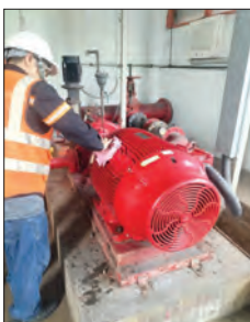
Photo 2.3 Cleaning Electric Motor
