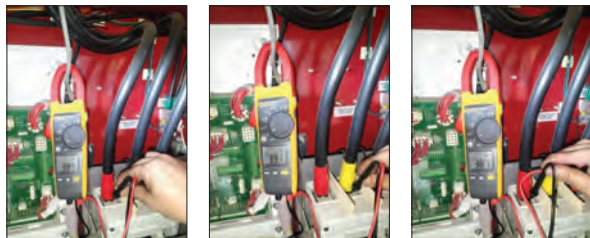
Photo 5.1.2 Checking the three-phase voltage of the fire pump electric motor control.
