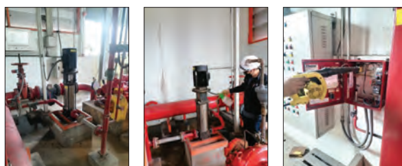
Photo 5.1.12 Clean jockey pump and jockey pump electric motor control cabinet.
