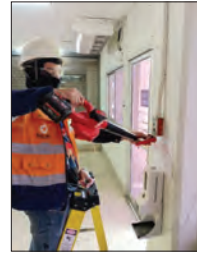
Photo 4.9 Check and Test Manual Pull Station.
