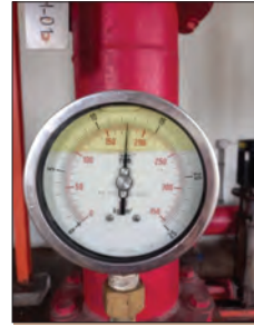
Photo 5.1.19 Pressure (Discharge 178 PSI).
