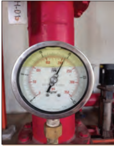
Photo 5.1.15 Pressure (Discharge 208 PSI).
