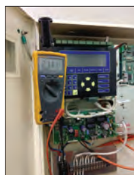
Photo 2.1.2 Check Backup Battery.
