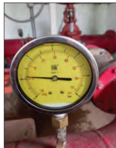
Photo 5.1.22 Pressure Suction 2 PSI.
