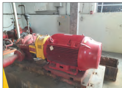
Photo 1.2 Main fire pump (Electric fire pump)
