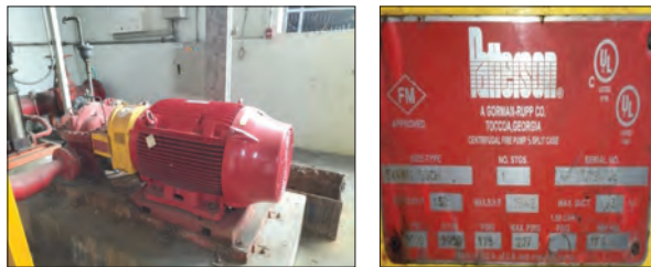
Photo 5.1.1 Electrical Motor Fire Pump.
