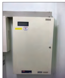
Photo 2.2.1 Fire alarm control panel in factory
