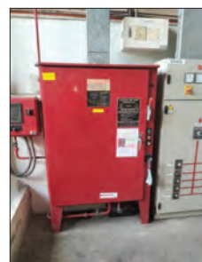
Photo 1.1 Fire pump control cabinet (Electric fire pump controller)
