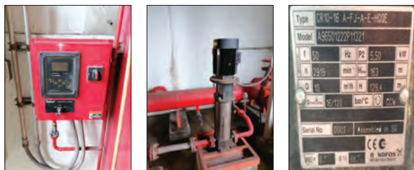
Photo 5.1.7 Jockey Pump and the control panel.
