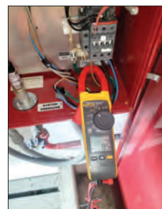
Photo 2.7 Motor Voltage and Current (Normal)
