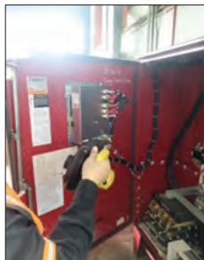
Photo 2.2 Cleaning Control Cabinet
