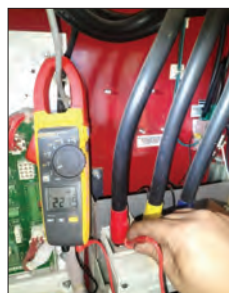
Photo 2.7 Motor Voltage and Current (Normal)
